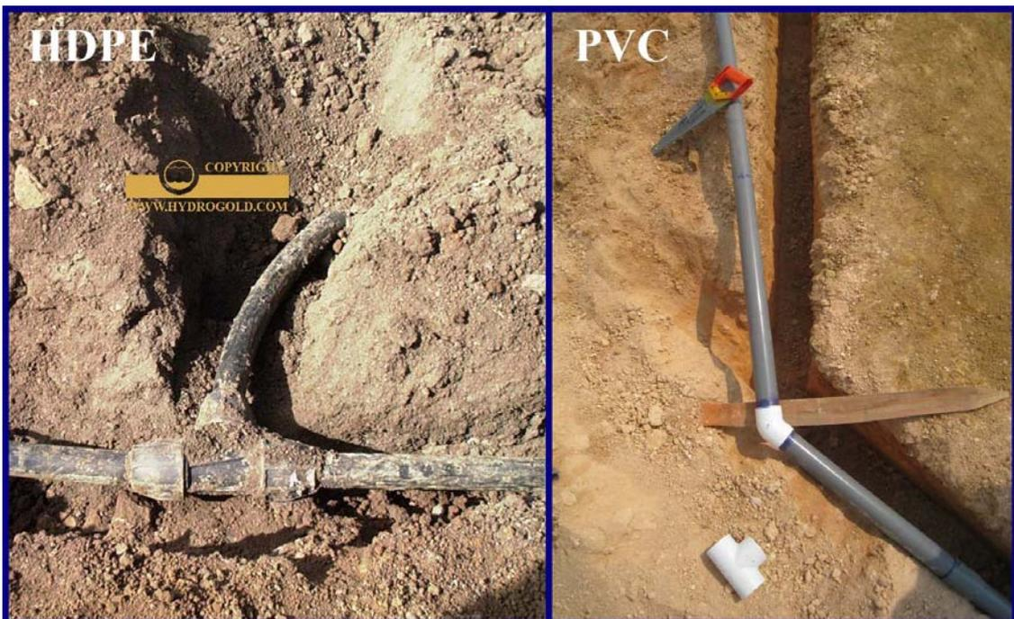
This HDPE pipe is severely bent and stress put on the joint. Despite such a poor installation, this joint will last many more years than the PVC elbow to the right.
