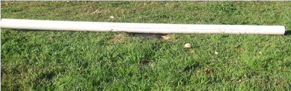
Then turn the pipe 90 degrees to ensure that the sprinkler is to grade in that direction also.
